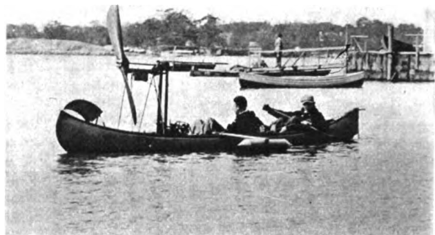
A Canoe Fitted with an Air-Cooled Motor Driving an Air-Propeller. While Not a Practical Mechanical Proposition Much Fun can be Derived from a Boat Thus Equipped
